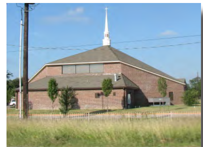
The newly constructed Emmanuel AME Church located off of Semlinger.
